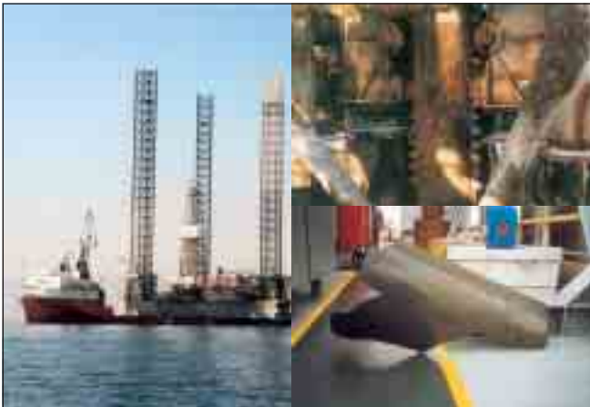
Picture 1+2+3 Bracing the legs of a rig for transport
