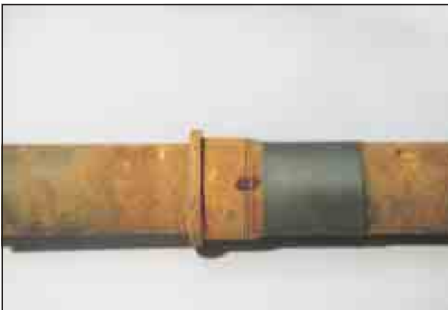
Picture 2 Repair of a primary shaft
