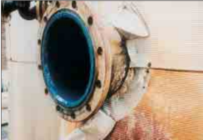
Picture 1 Entrance of CO 2 installation
