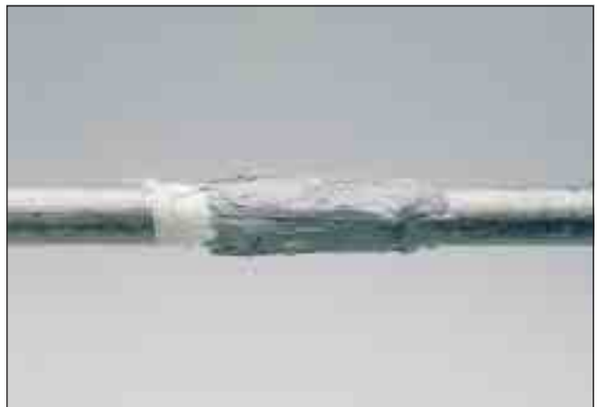
Picture 4 Emergency repair of pipes
